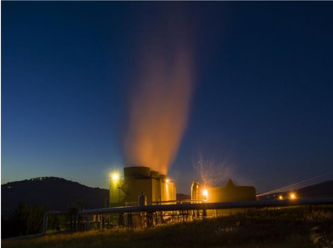
Combined biomass and geothermal plant in Cornia, Italy
