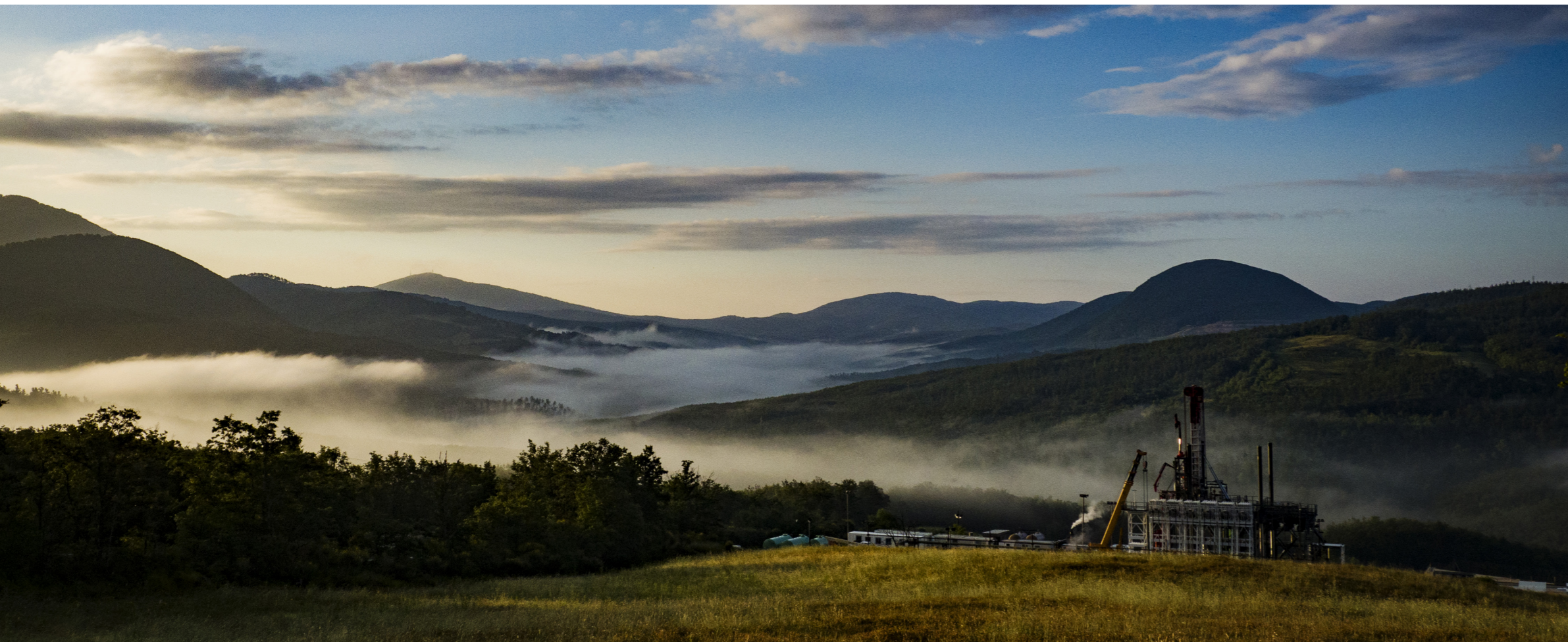
Photo: Combined biomass-geothermal power plant "Cornia 2", Italy
